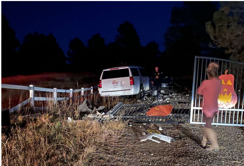
Our front gate after the third encounter with a vehicle
